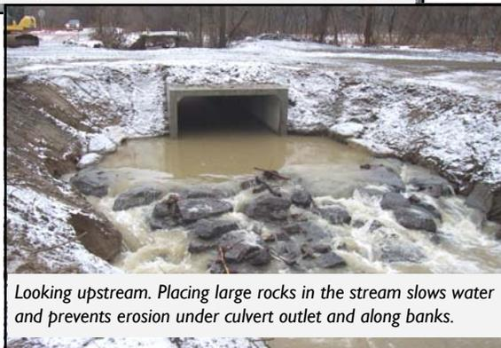
Looking upstream. Placing large rocks in the stream slows water and prevents erosion under culvert outlet and along banks.
