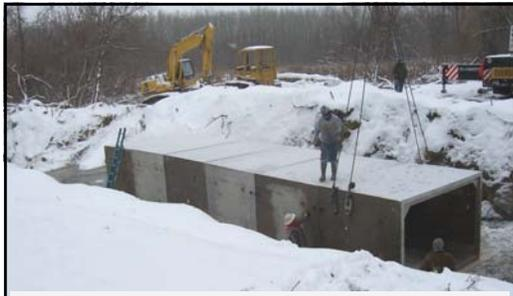
Contractors place modular culvert sections with a crane
