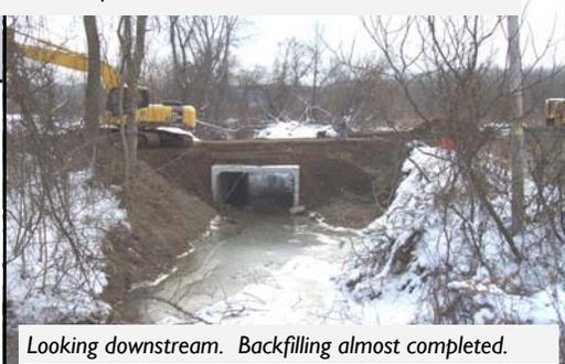
Looking downstream. Backfilling almost completed.
