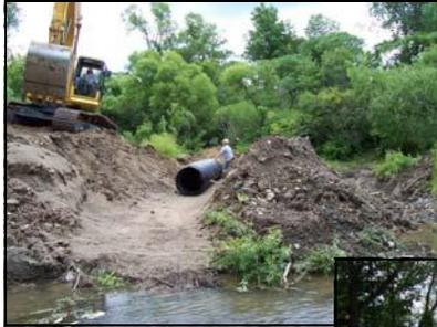
**Rockville:** Construction is progressing on the trail crossing at the Rockville Lake outlet. A culvert was installed in the present-day outlet and covered with 1,800 tons
