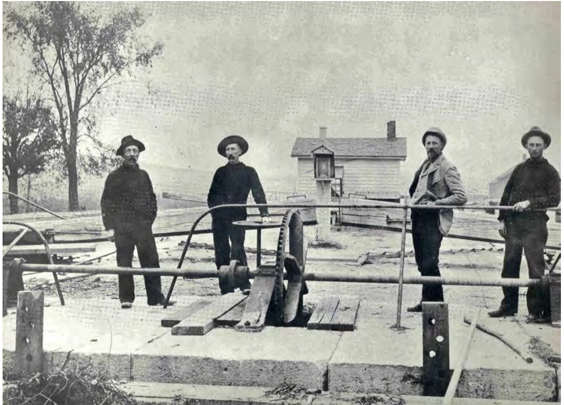
Lock Tenders at Erie Canal Lock #61, Macedon
